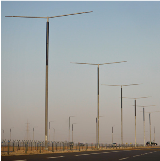
Ghayathi Highway, Abu Dhabi, U.A.E. Worldwide first 100 % solar and 100% off-grid highway lighting
